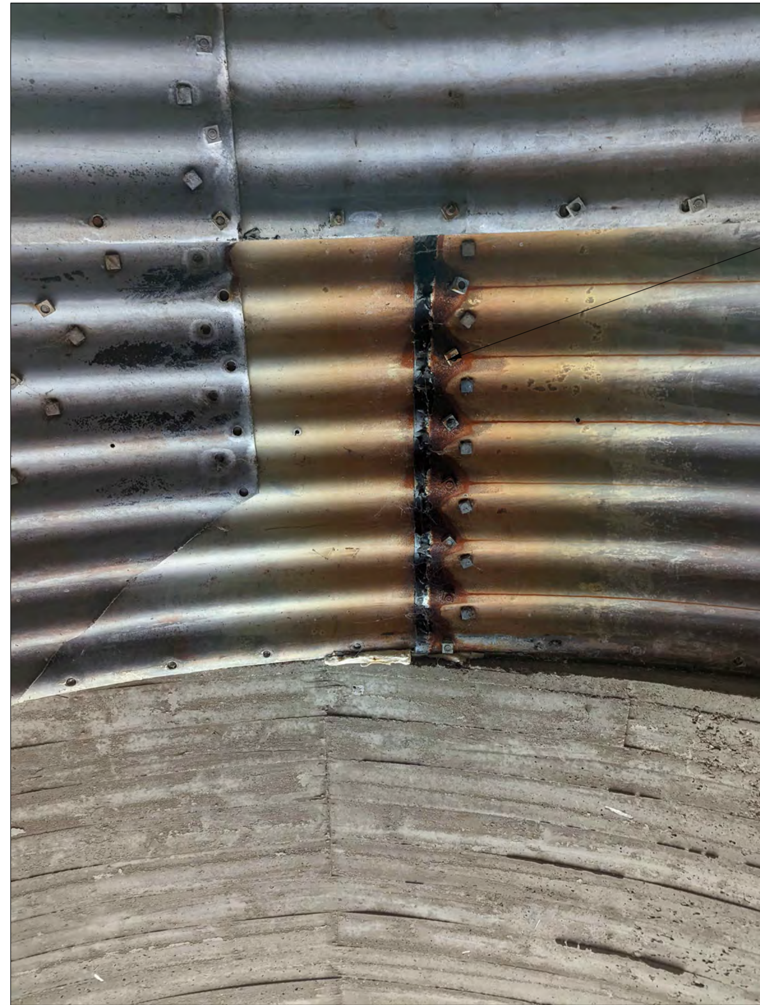
TOP OF ARCH AT END OF STRUCTURAL PLATE
