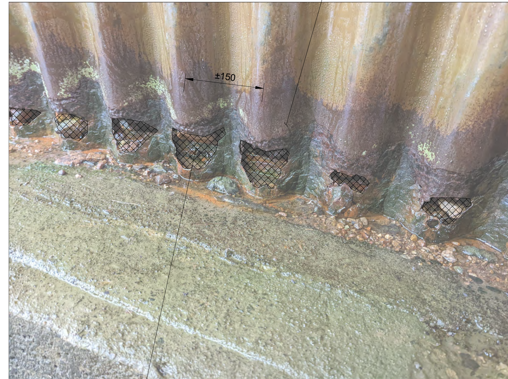
PERFORATIONS AT BOTTOM OF STRUCTURAL PLATE (EAST SIDE)
